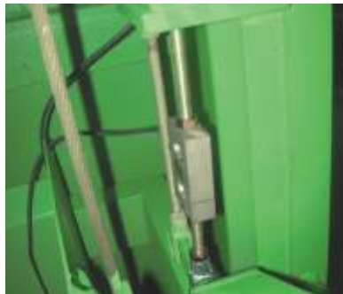
Aggregate Weighing system
